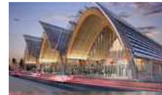
10 Mactan-Cebu International Airport
